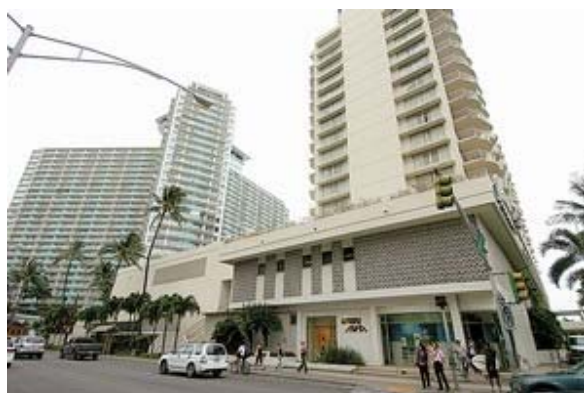
The former Yacht Harbor Tower adjacent to the Ilikai is under renovation and is expected to soon reopen as a luxury Edition hotel.
